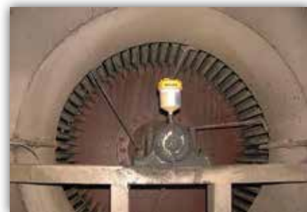
Streamliner V installed on a blower fan
