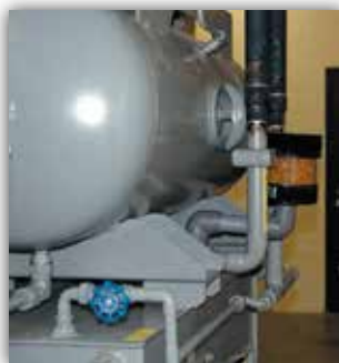
Watchdog Breather installed on a hydraulic reservoir
