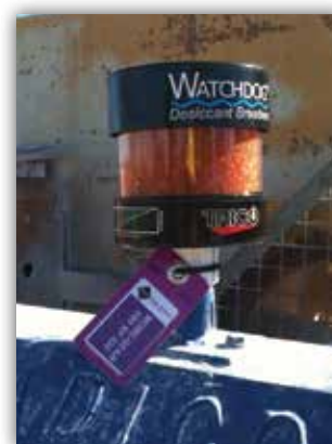
Spectrum Tag on a Watchdog Desiccant Breather
